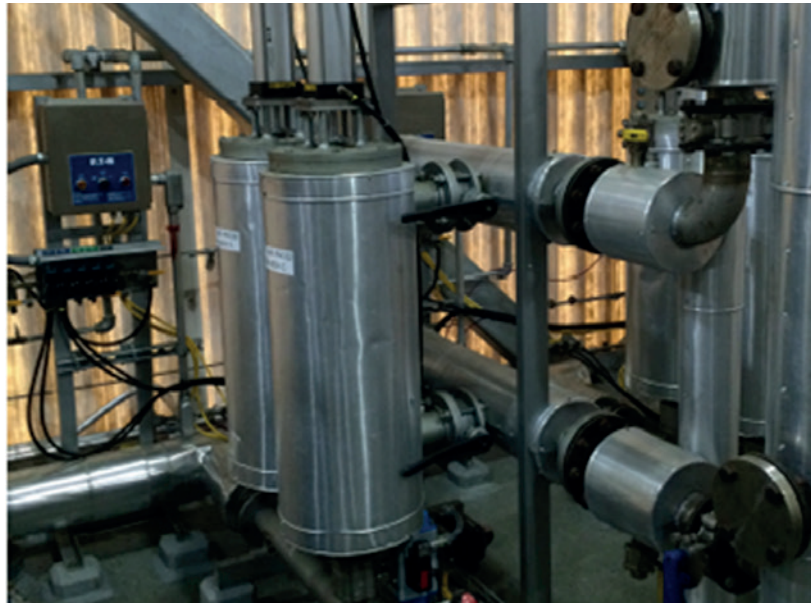
Eaton's series of mechanically cleaned filters work well with highly viscous, abrasive materials or liquids with heavy amounts of particulate.
