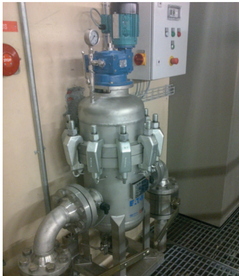
Eaton Model 2596 automatic self-cleaning strainer (version for pressures up to 1,450 psi (100 bar)).
