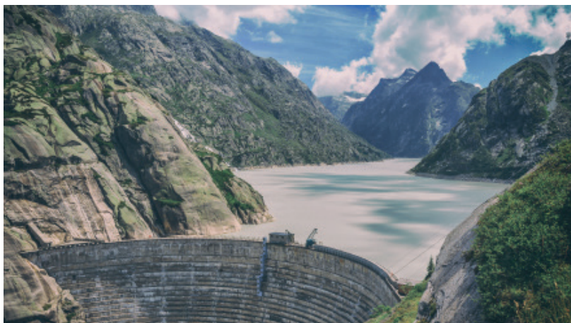
The Kraftwerke Oberhasli AG power plant (KWO) can generate energy on demand at any time using water dammed in the Grimsensee, 1909 m above sea level. (Image: Shutterstock)
