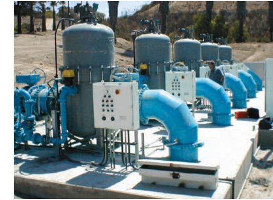
Five 24" Eaton Model 2596 strainers with backwash assist pumps installed at a potable water treatment plant.
