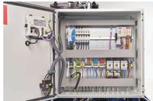
Web-enabled control unit with touch panel and USB interface
