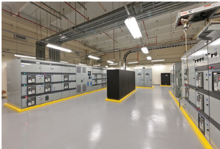
Figure 1. MCCBs protecting critical equipment at the Eaton Bluegrass Data Center in Bluegrass, KY.
