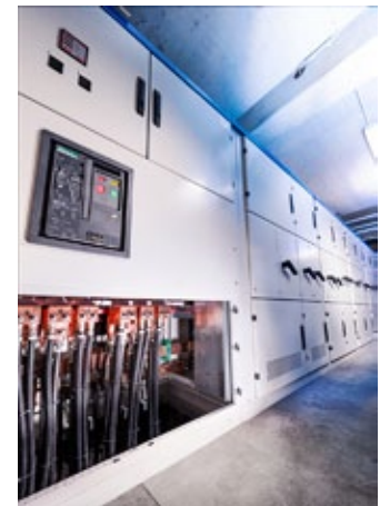
Today, Eaton's xEnergy can provide as much as 5,000 A via a single feeder section
