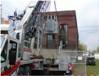
Rigging a new GSU transformer
