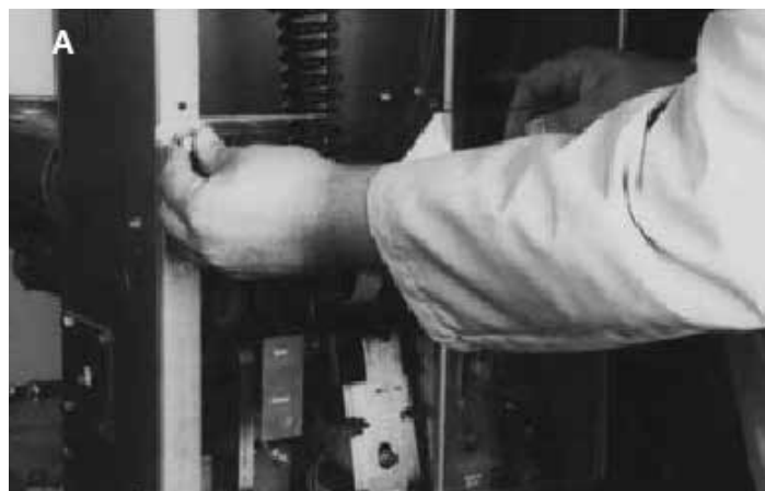
Figure 34. Attaching CloSure test tool at hole "A".
