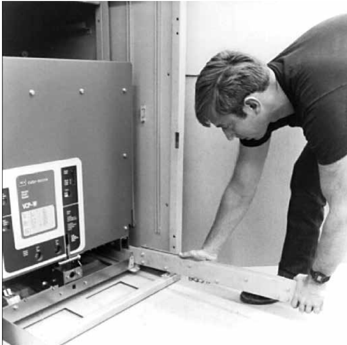
Figure 15. Engaging extension rails in a lower circuit breaker compartment.
