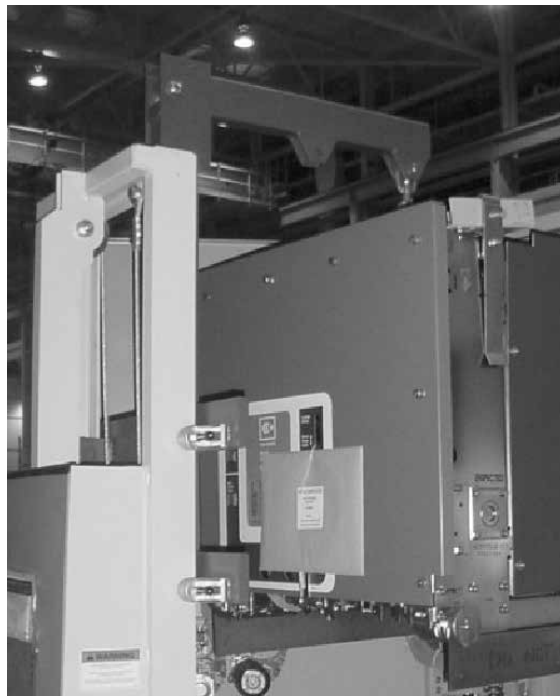
Figure 12. Lifting and setting the breaker in the housing.
