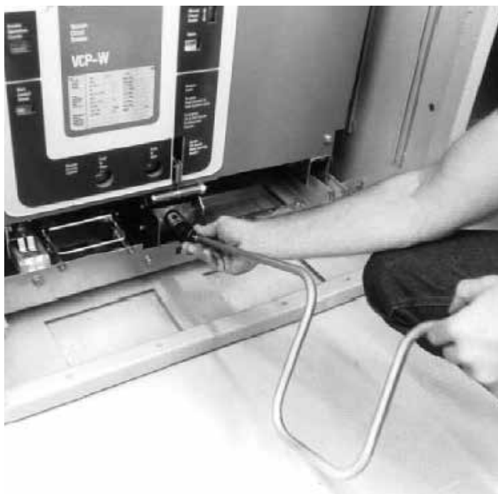
Figure 18. Engaging levering-in crank.
