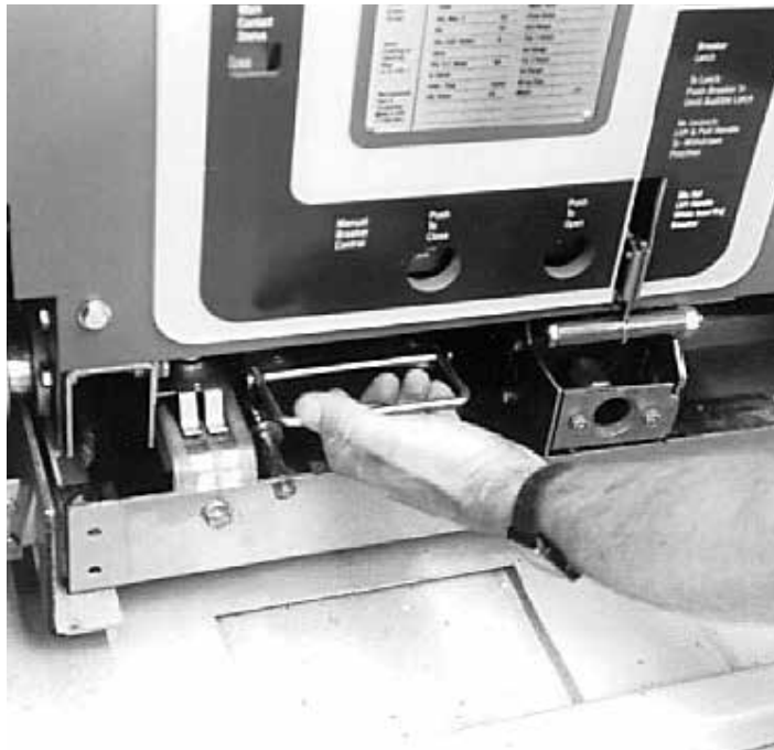
Figure 17. Pulling secondary disconnect cage to engage secondaries in TEST position (old version shown). New version will have BPI pan with automatic secondaries.
