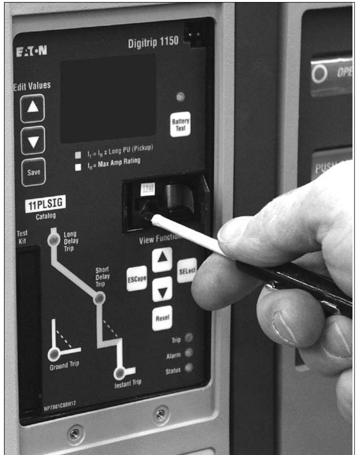
Figure 3. Installation of the rating plug and mounting screw
