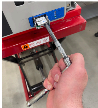
Figure 11. Manual racking.
