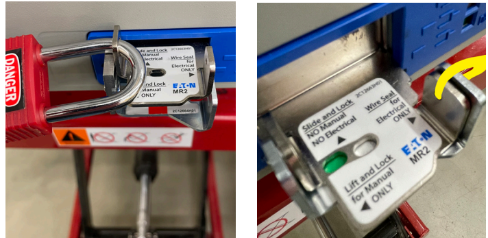
Figure 8. MR2 racking prevented (manual racking allowed).
