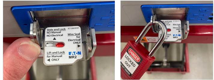
Figure 7. Padlock slider permissive actuated (no racking allowed).
