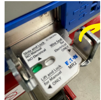
Figure 9. Door lifting is blocked (MR2 racking allowed).
