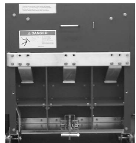
5/15 kV Manual G&T Device shown with Lower Terminals Grounded
