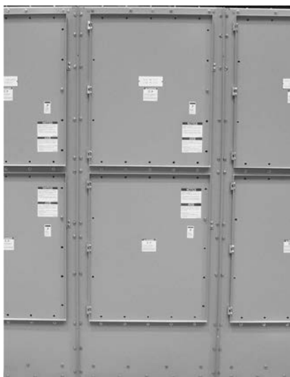
Rear View 5/15 kV VCP-W Arc-Resistant Switchgear
