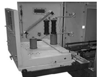
Fuse Drawer— Shown Fully Withdrawn
