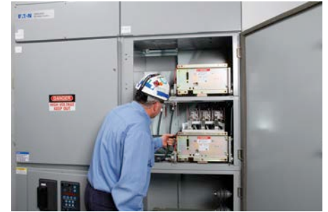
Arcflash Reduction Maintenance System (ARMS)
