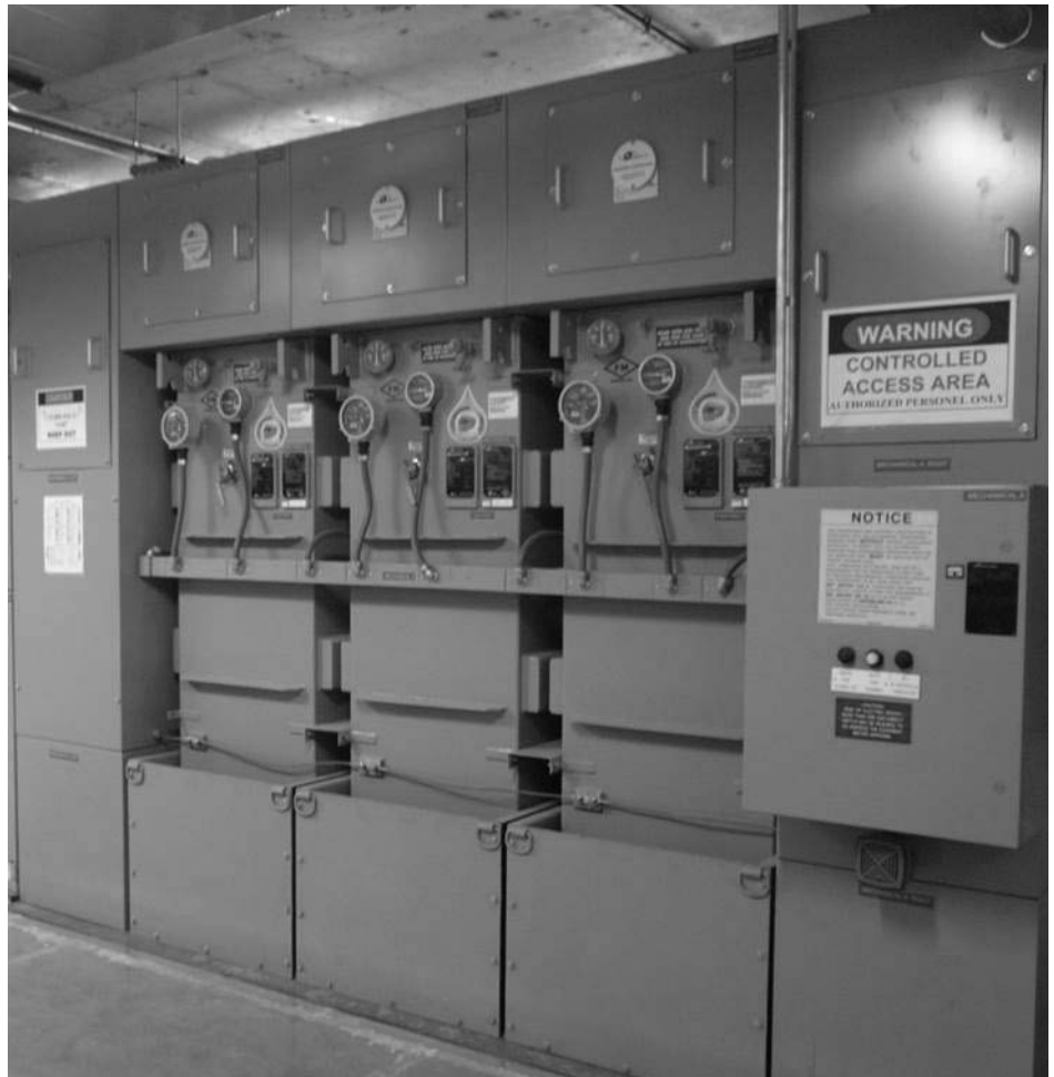
Triplex Indoor Power Center
