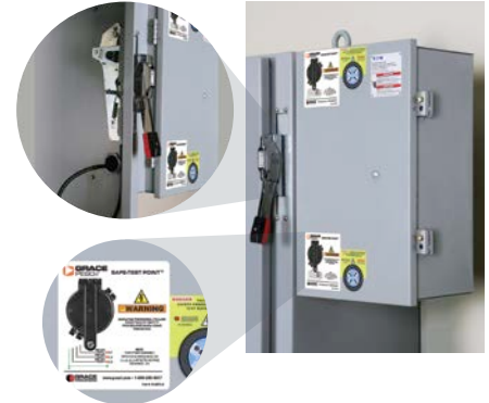
OLI Switch Integrated onto Disconnect Enclosure
