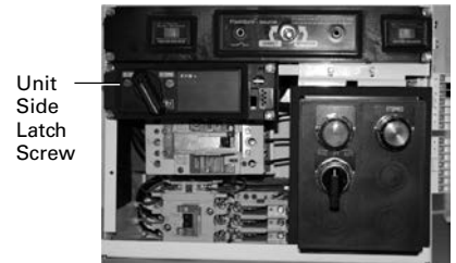
Freedom FlashGuard Unit Wrapper Side Latch
