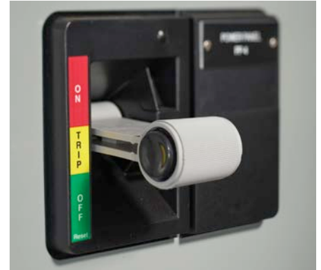
Circuit Breaker Handle Mechanism
