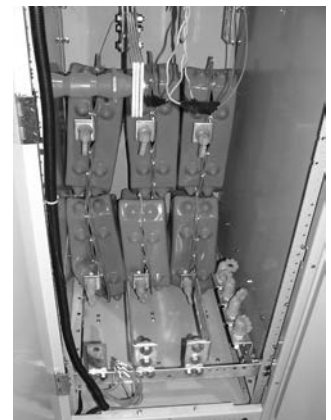
Grounding Balls and Covers
