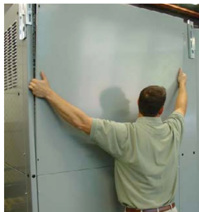
Removing the Upper Side Cover, Lifting Brackets can be Seen at the Top
