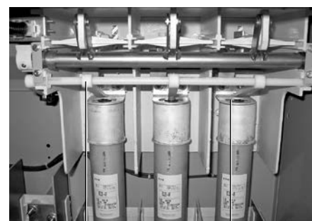
Blown Fuse Indicator Operating Arm (Optional) Fuse Fault Indicator
