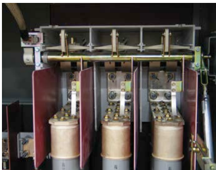
Blown Fuse Indicating Device
