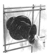
Remove forms. Then end caps may be replaced to protect sleeve from dust and debris until conduit penetration is made. At that time remove caps and wipe the sleeve clean.
