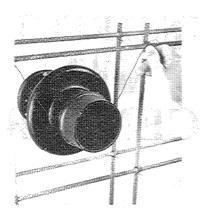
4. Before final form is positioned, place second end cap on sleeves. Check to determine that cap is properly inserted.
