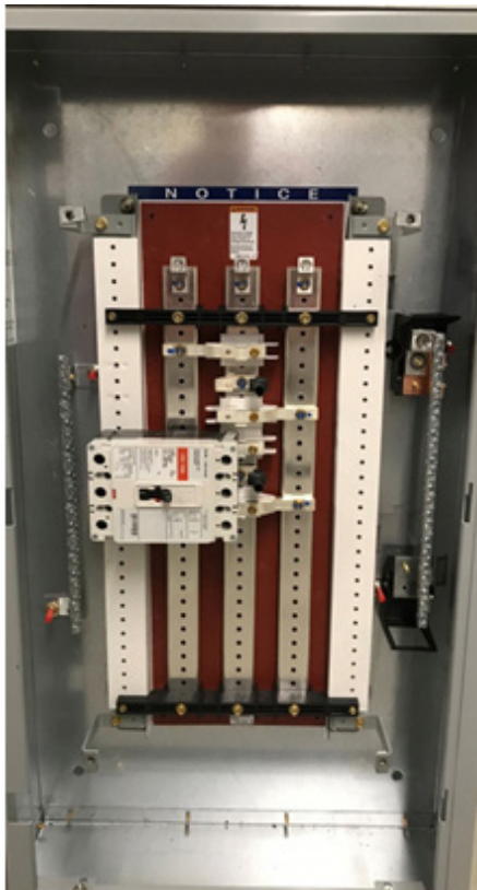
Figure 4. PRL3a with connector kit installed.
