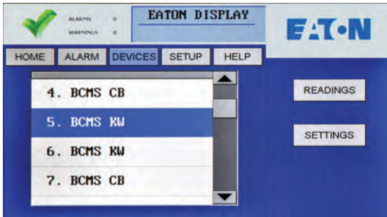
Figure 26. Readings: BCMS KWH (Part 1)
