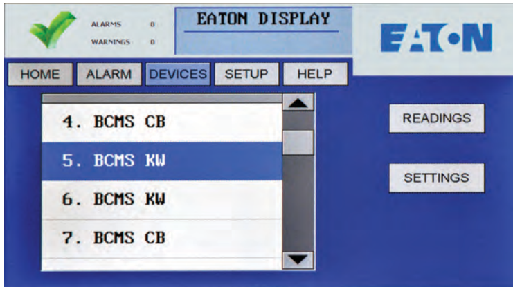
Figure 33. Find the Circuits in an Alarm Condition
