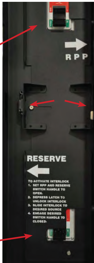
Figure 21. Mechanical Transfer Interlock
