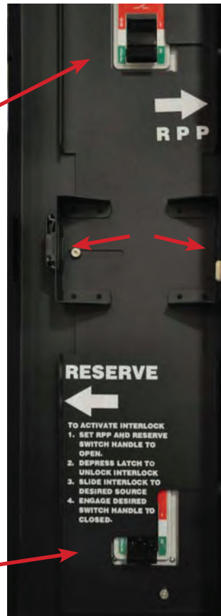
Figure 10. Mechanical Transfer Interlock
