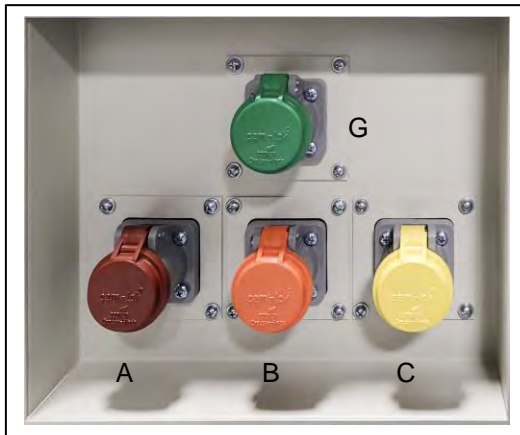
Figure 45. Optional Cam Locks for Second Power Source
