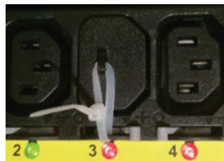
Cap secures in place with cable tie
