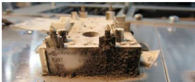
Close-up photo of an IGBT inside a power module which overheated due to effects of dirt and dust collection overtime.
