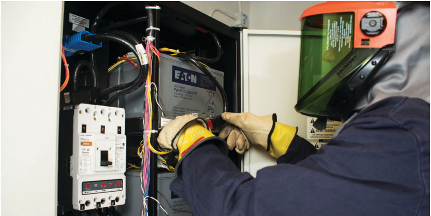
Appropriate personal protective equipment is essential when working on batteries or any UPS equipment
