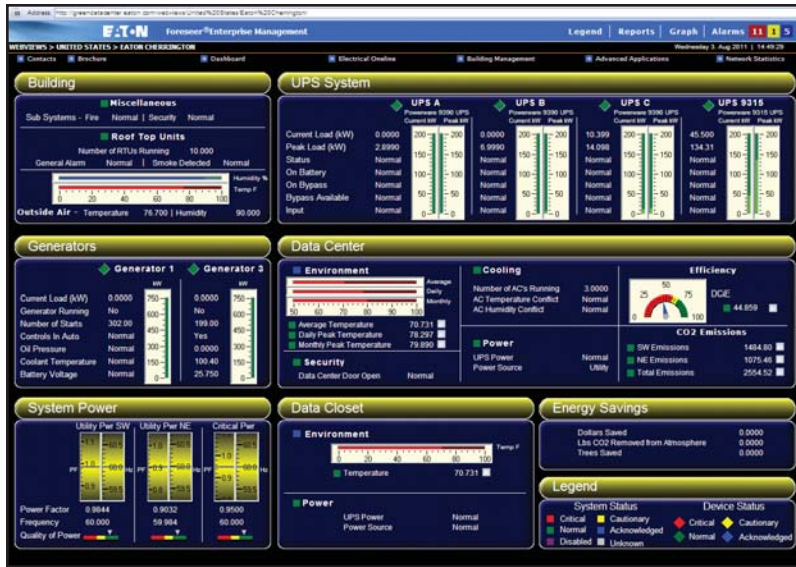
Figure 3. Eaton's Foresee Enterprise Monitoring software works in conjunction with building management systems (BMS) to provide comprehensive and "real time" view of the electrical, mechanical, life safety and security systems.
