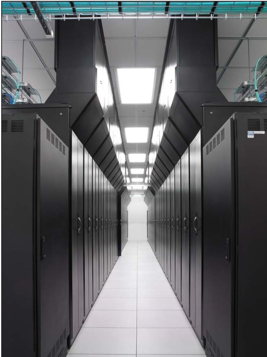
Hot exhaust air is removed from the server enclosures via HCS chimneys located on the top rear of the racks and is then directed back to precision cooling units (the CRACs) by way of a ceiling plenum.
