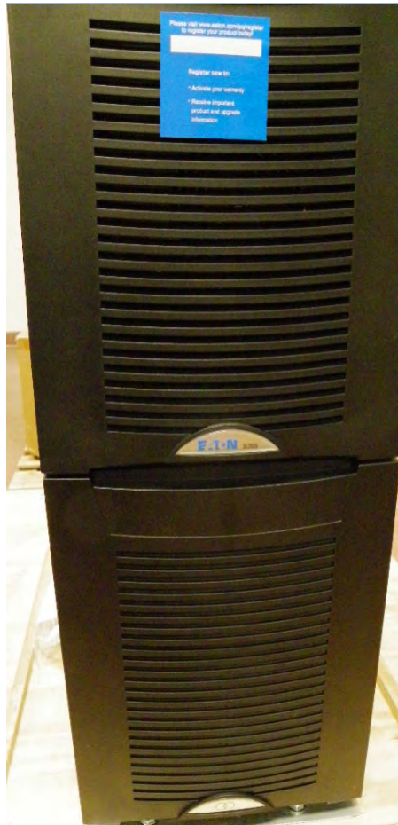
Figure 25. Battery Cabinet Front Dress Panel Reinstalled
