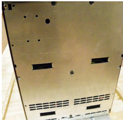
Figure 24. Reinstalled Dead Front
