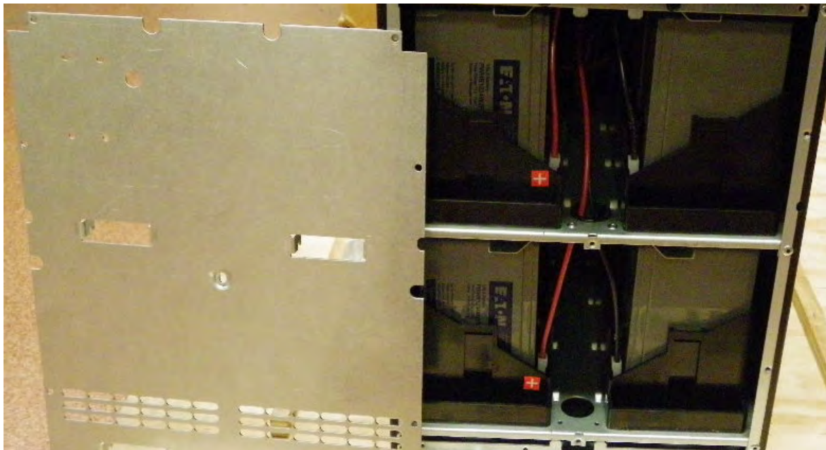
Figure 5. Battery Dead Front Removed
