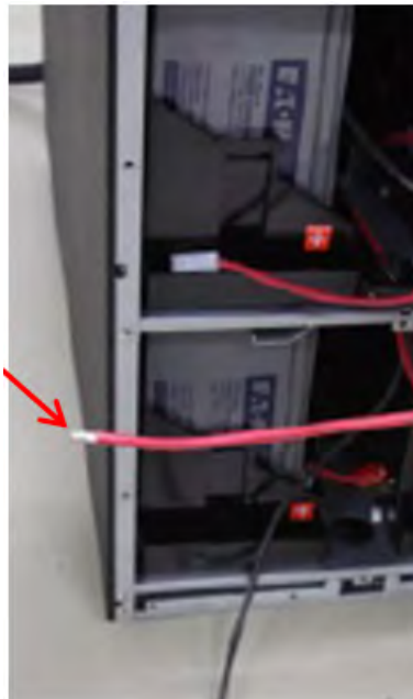
Figure 15. Strip 1/4 Inch of Insulation
