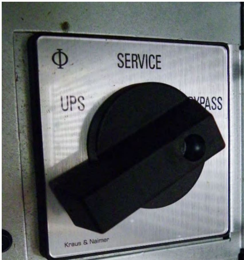
Figure 1. Bypass Mode (UPS mounted Maintenance Bypass Switch located at the rear of the unit)
