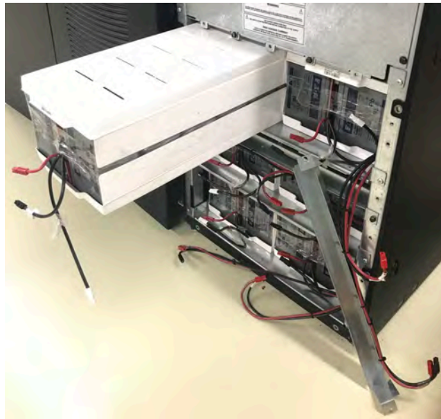
Figure 8. Remove an old Two-Row Battery Tray
