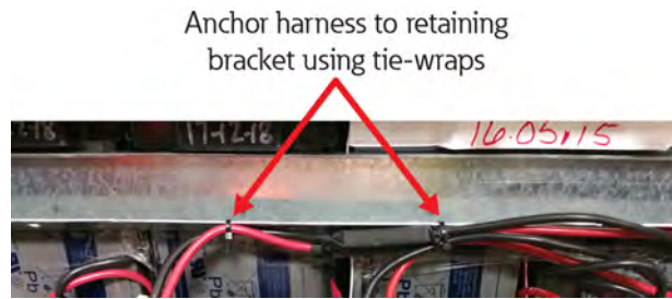
Figure 13. Anchor Battery Harness to Battery Retaining Bracket
