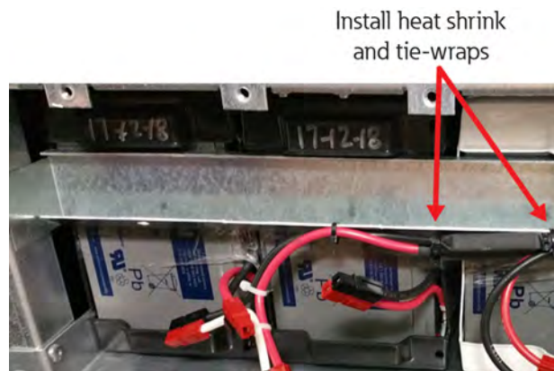
Figure 12. Install Heat Shrink Tubing and Secure Using Tie-Wraps
