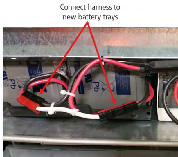
Figure 14. Connect Battery Harness to New Single-Row Battery Trays
