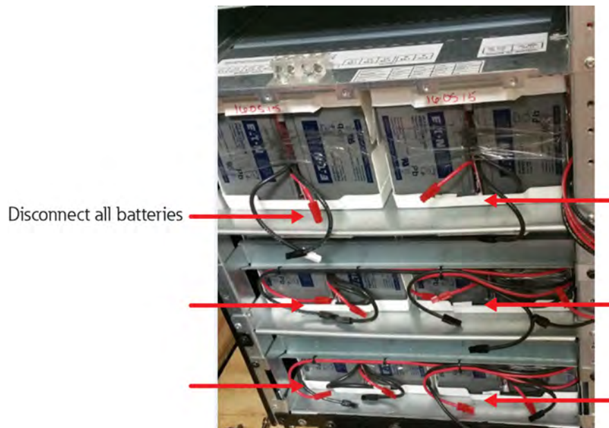
Figure 6. Disconnect All Battery Trays
