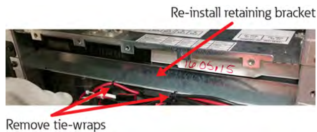
Figure 10. Re-install Battery Retaining Bracket and Remove Tie-Wraps
