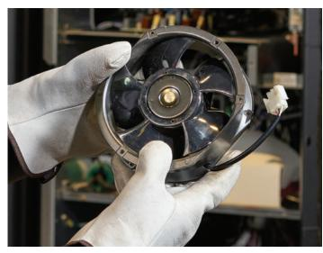
Fans are one of the few UPS components that are mechanical in nature. They wear out over time and eventually need to be replaced, usually after six or seven years of use.
