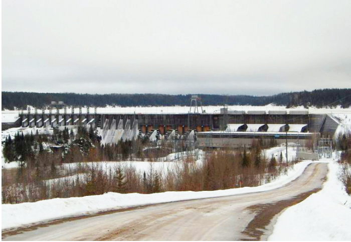
Existing station prior to electrical upgrades
