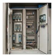
The Eaton SLX9000 inverters are communicating with the PLC via CANopen; motor starters are connected to the PLC via SmartWire-DT.
