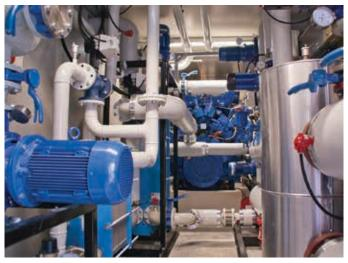
The system supplies electricity to the factory from the methane-fueled motor and uses the residual thermal energy to process heat transfer oil.
