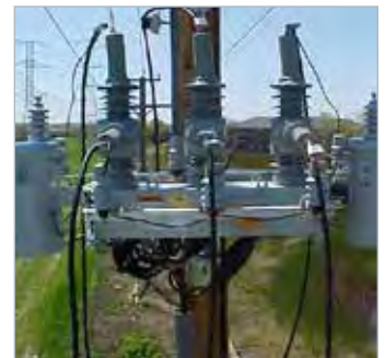
NOVA™ three-phase recloser and control
