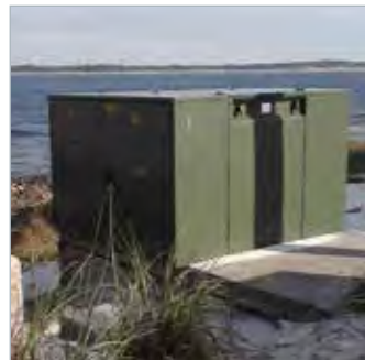
Smart VFI pad-mounted switchgear
