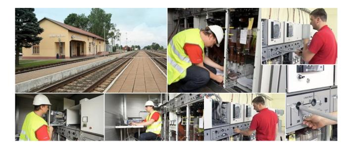
Eaton Xiria ring main units and SVS 08 series switchboards for the project. Another key factor was the very compact construction of these products, which not only made them easier to handle, but also meant that they could be accommodated in smaller buildings with lower construction costs.
