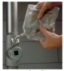
Fig. 3 Cement type of sealing compound in a burst pouch configuration.
