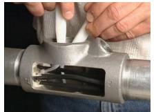
Fig. 13 Figure showing the damming and conductor separation required for cement type of sealing compounds.
