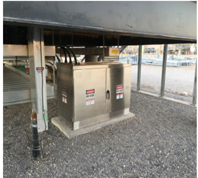
Fig. 13. Completed snubber installation at EEC-11.
