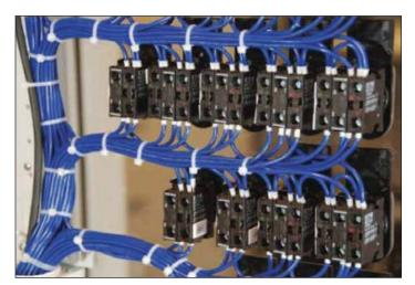
Figure 2. Additional control panel construction time is required when wiring is bundled to door-mounted devices because wires must not restrict opening and closing the door
