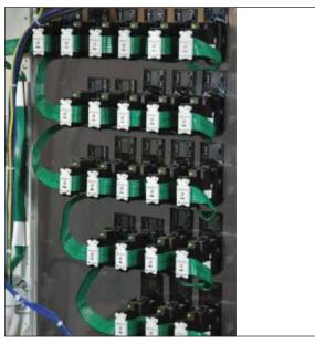
Figure 6. Device-level wiring systems use flat multiconductor cables to connect components, replacing bulky wiring ducts found in conventionally wired control panels
