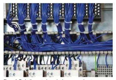
Figure 3. Typically, control panels change over time to accommodate wire tracing, configuration/design modifications, the addition or removal of control or electrical components, or tapping into the control power supply
