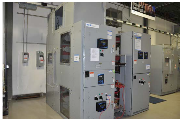
Medium-voltage switchgear
