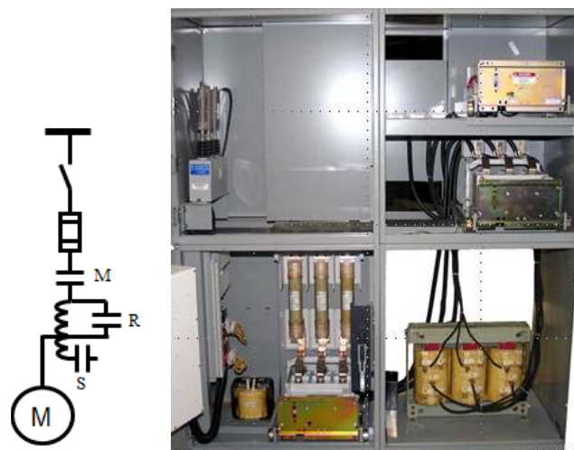
Fig. 8. One-line diagram and photo of a typical autotransformer starter
