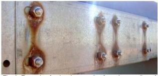
Fig. 3 Example of galvanic corrosion from the coupling of stainless steel plate with mild steel hardware. [5]
