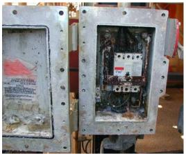
Fig. 11 Severe corrosion of a bolted enclosure.
