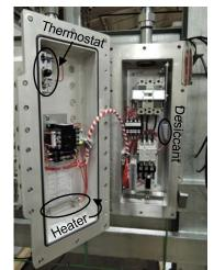
Fig. 13 Enclosure with heater, thermostat and desiccant pack for moisture control.
