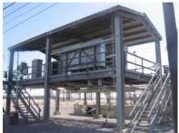
Fig. 16 Use of shelters can help to minimize environmental exposure leading to reduced corrosion. Reprinted, with permission, from [17]
