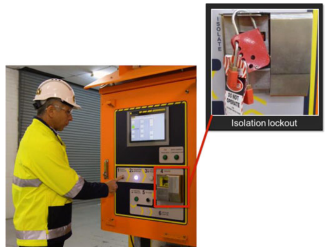
Fig. 5. FIS user interface panel with isolator lockout switch and hasp for personal isolation padlock(s).
