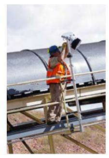
Fig. 4: Telescoping light poles being installed in mine site conveyor system
