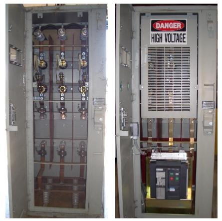
Fig. 3. Above left is a photo of the existing primary fused load-break primary switch for each substation with the fuse holders still in place. Above right is modified assembly after modification, with fixed mounted mini-vacuum circuit
