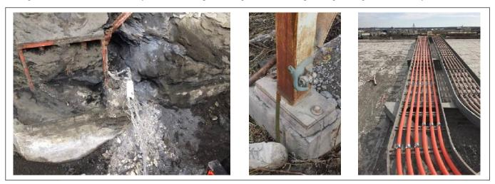
Fig. 7. As found ground connections compromised or severed grid at left and center, 5kV existing replaced cable at right.
