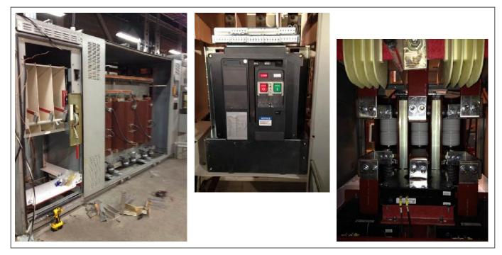
Fig. 4. Existing primary switch at left, retrofitted with new vacuum circuit breaker at center and current transformers at the rear of the breaker at right.
