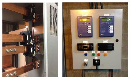
Fig. 5. Transformer secondary bus with new current transformers at left, new protective relay cabinet at right.
