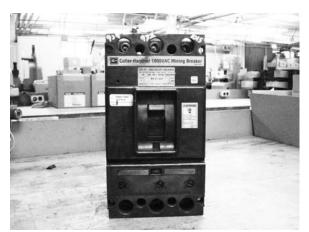
Figure 3. Eaton Manufactured Mining Breaker with Proper Identification and Labeling; Successfully Passed Testing Sequence
