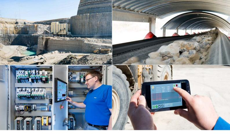
The XC-202 modular PLC controls our processes in the buffer silos. Thanks to the PKE motor-protective circuit-breakers networked via SmartWire-DT we can prevent an overload of the drives," says Gerd Bader, plant electrician at bmk
