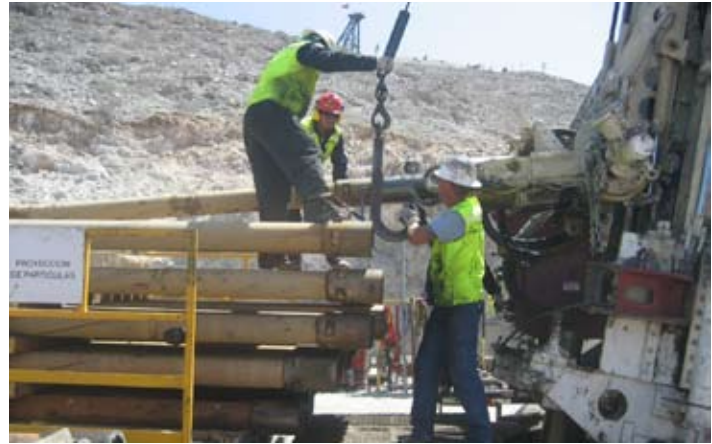
Workers add another piece of drill pipe to the Schramm T130XD.
