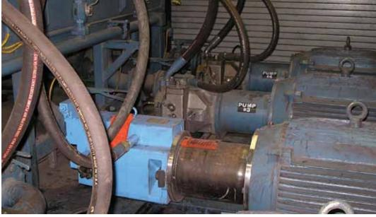
Because Gerdau Ameristeel's walking beam furnace needs to operate continuously at peak performance, its power unit consists of a series of four 250-ccm piston pumps, three of which are operational and one on standby as a "hot spare." Oversized shaft and shaft bearings enable Eaton's Hydrokraft PVX pump to provide the water glycol-based power unit with reliable operation and long life.
